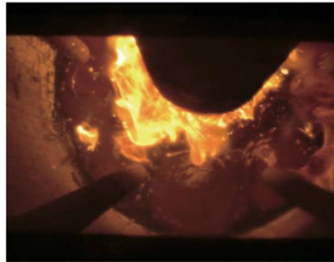
(b) Overhead view of the condition of the CCIM furnace
