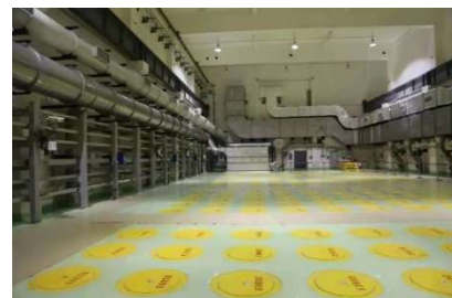
Sampling (top), pouring (middle) and temporary storage (bottom) https://www.caea.gov.cn/n6760338/n6760342/c6831032/content.html
