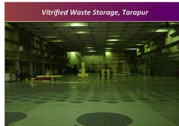
Interim storage facility for radioactive vitrified waste products at Tarapur.
