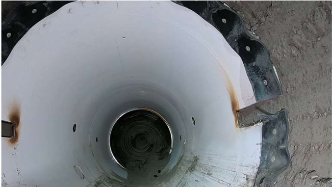
Thickness of cementitious filling grout between 2 and 22 cm (mean value = 8 cm)
