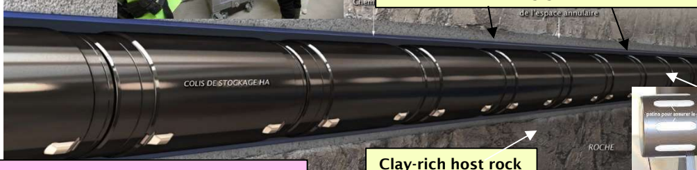
Micro-tunnel with steel sleeve
