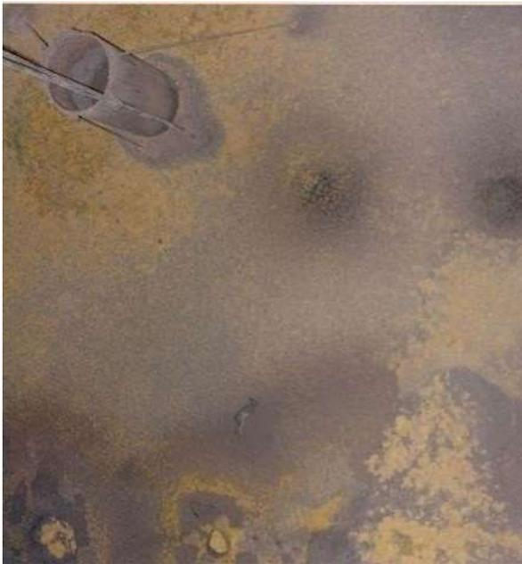
Sludge and debris – Tank SX-114
