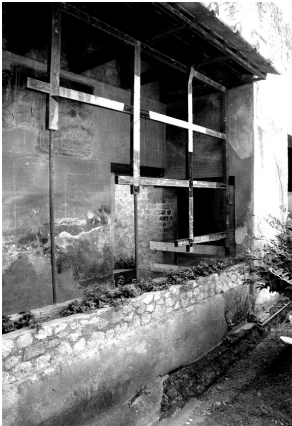
Charred remains of the glass partition in the eastern portico of the uiridarium of the Casa dell'Atrio a Mosaico (IV, 1-2) at Herculaneum
